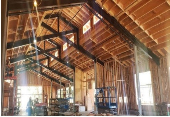
Building in Progress
