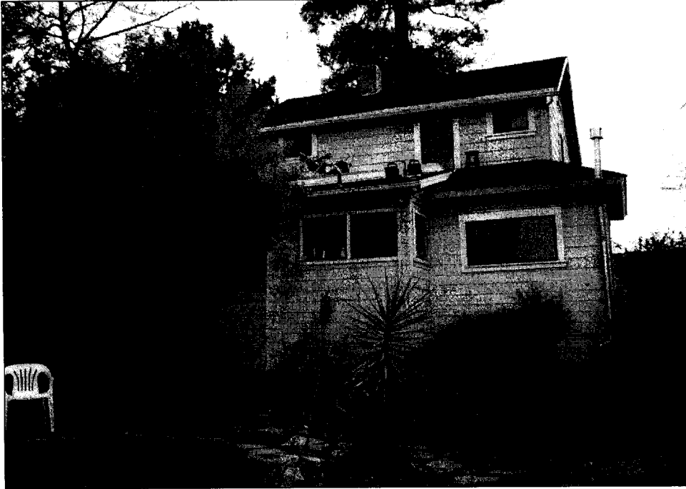
Figure 1. Main house, looking northeast at west elevation, 12/7/05.
