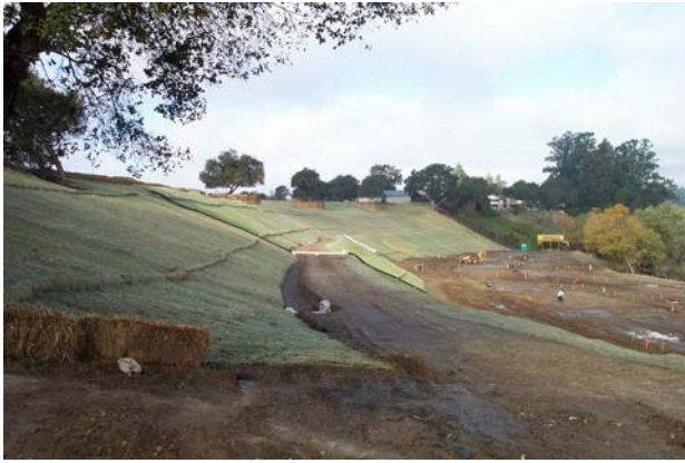
Picture 2. Effective use of erosion control blankets placed on a steep slope. Seed was spread prior to placing the blankets.
