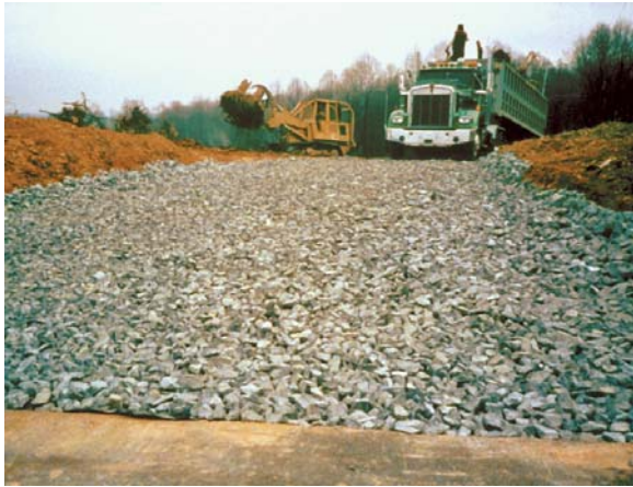
Picture 7. Rocked Construction Entrance.
