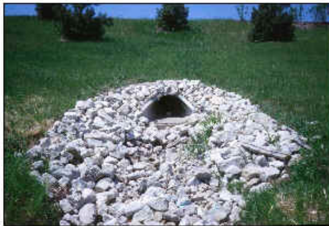
Picture 9. Rock Energy Dissipator.
