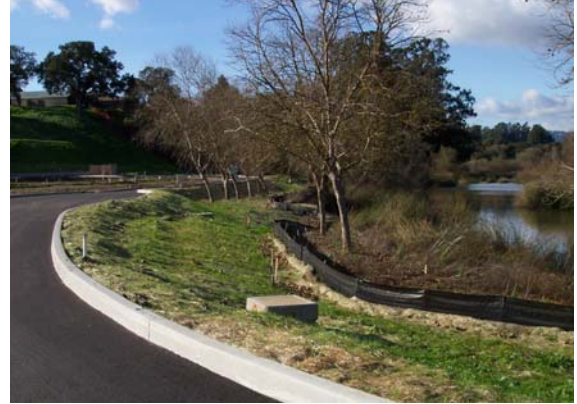
Picture 5. Use of silt fencing and straw rolls for sediment protection of the adjacent lake.
