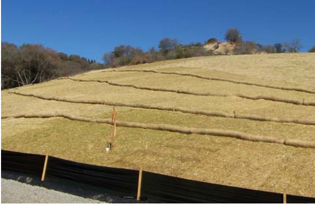
Picture 4. Use of straw rolls on a slope with a silt fence at the bottom of the slope. Note: This slope has also been seeded, and the steeper portions have been covered with erosion control blankets.
