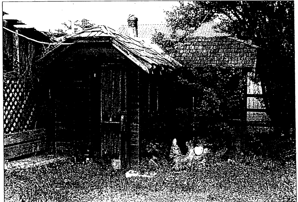
Figure 9. Sauna/Shower, looking northeast at west and south elevations, 3/26/07.
