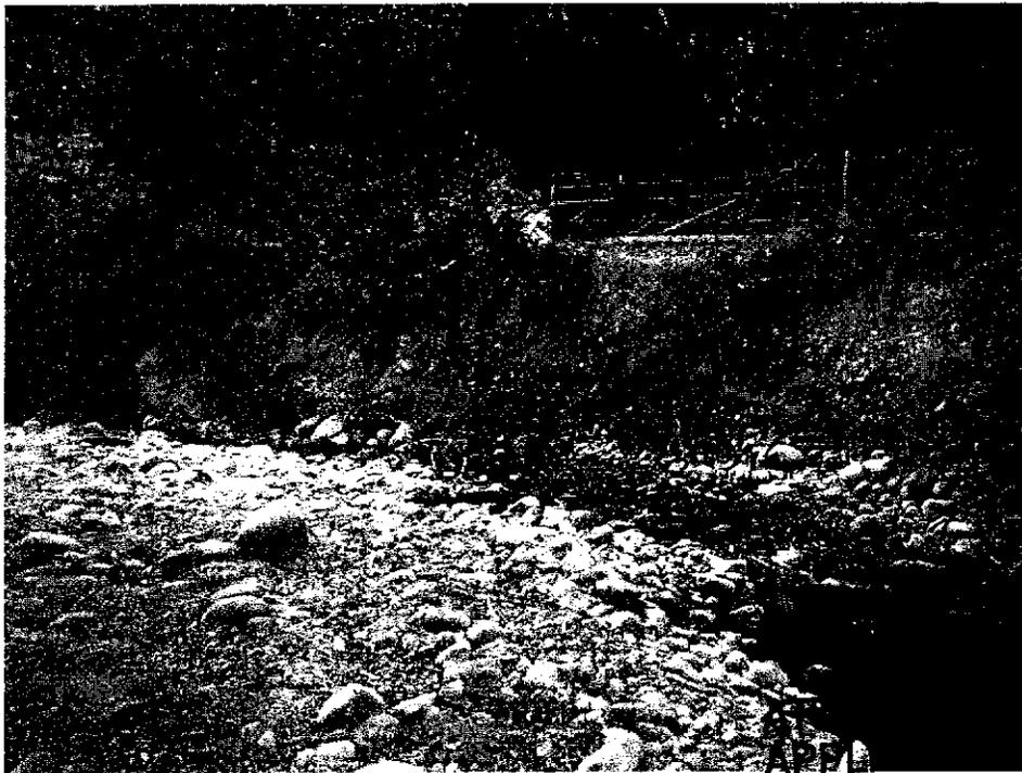
**Photograph 6 State Action Area. View of creekbank roadway embankment failure from creekbed showing exposed alluvial substrate and road fill material.**
