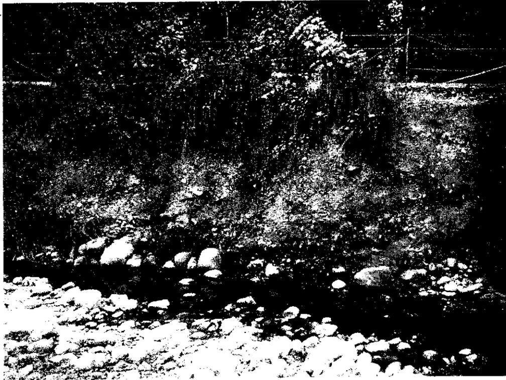
**Photograph 9. State Action Area. View of failed creekbank/roadway embankment below Hihn's Mill Road showing alluvial substrate and remaining patches of riparian vegetation on upper part of bank.**
