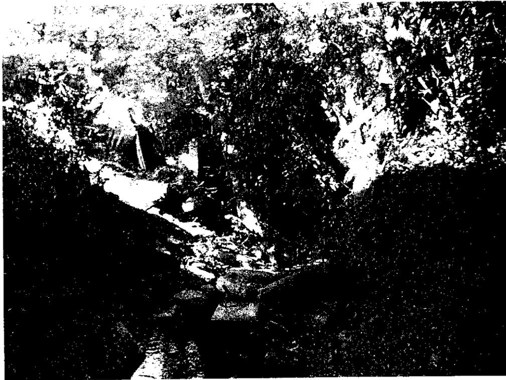
**Photograph 2. County Action Area. View of slide looking up stream with riprap debris in channel.**
