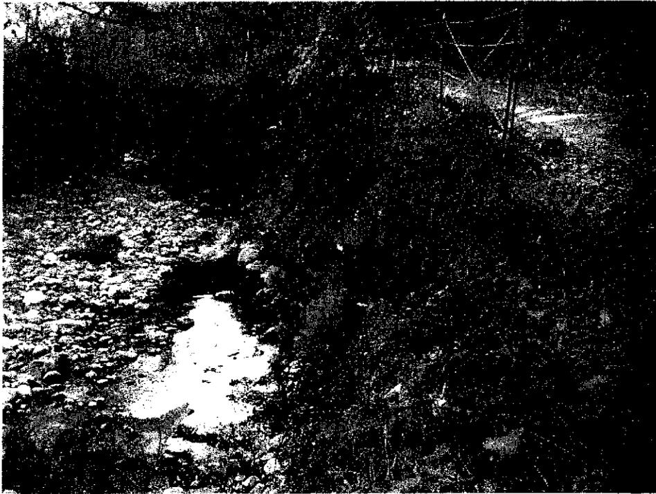
**Photograph 5. State Action Area (P.W. #2619). View of creekbank roadway embankment failure on Hihn's Mill Road adjacent to the East Branch of Soquel Creek.**
