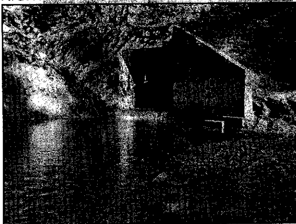
LEFT: E.C. 2.95 box culvert outlet and scour pool during low flow RIGHT: Culvert outfall during storm flow
