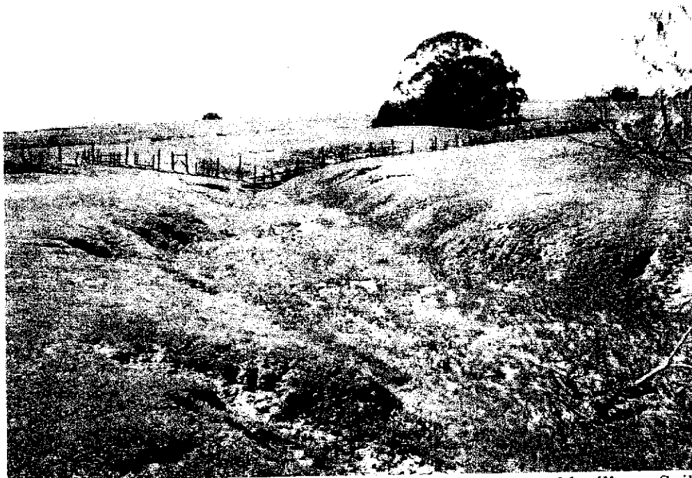
FIGURE 1. The lower fill site in 2000, looking downstream from the old willow. Soil has since eroded from the channel bed, therefore the repaired channel bottom will be lower than it was in 2000. The banks will be rounded and the channel bottom will be flat, as in this photograph.
