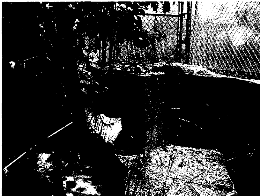
Concrete headwall with 18" RCP inlets
