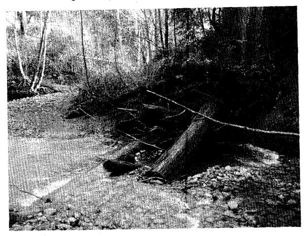
This photo shows an example of how a rootwad was cut and a portion of the stem preserved. This project will maximize the length of stem preserved.
