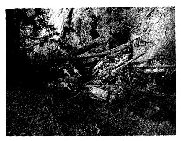
This photo shows an accumulation of large woody material that was mildly threatening the road. The yellow arrows point to a few key pieces that were cut to encourage a clear path for the creek while preserving the large woody material against the eroded slope.
