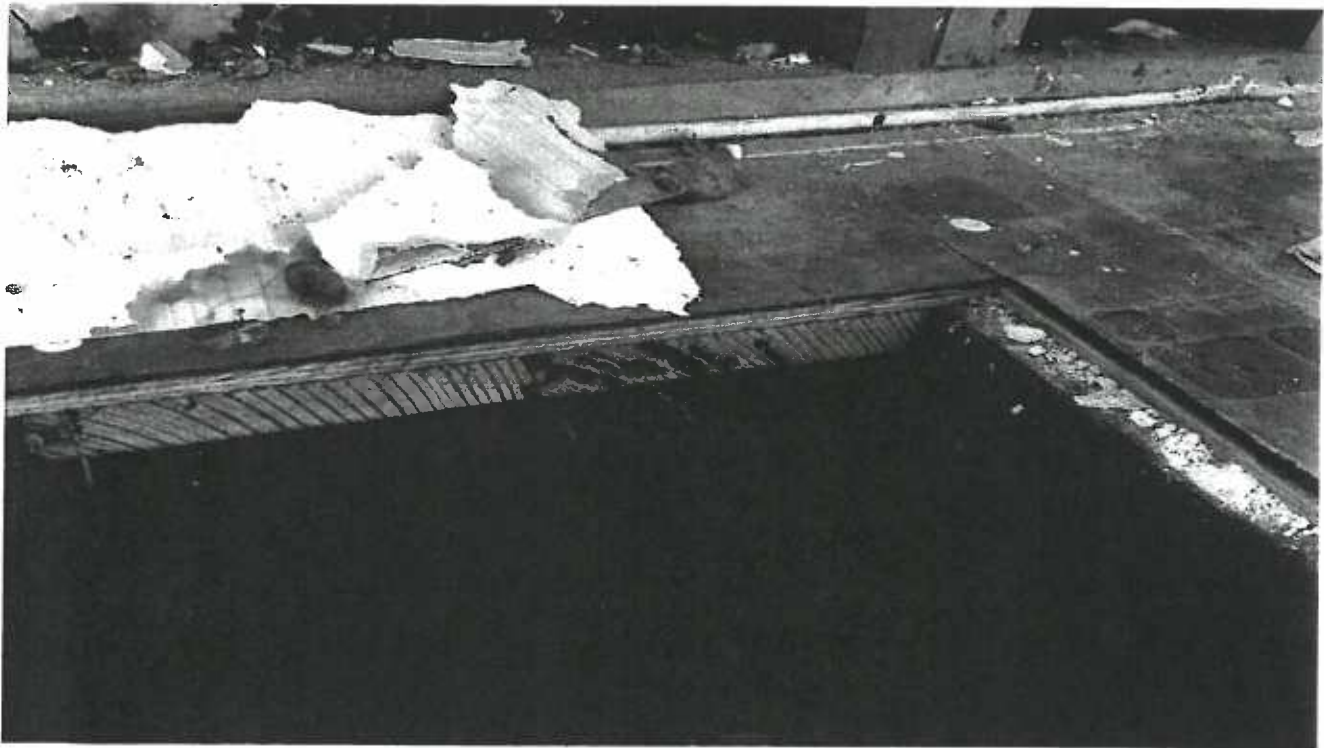
Figure 12. Heavy termite infestation and damage at floor deck
