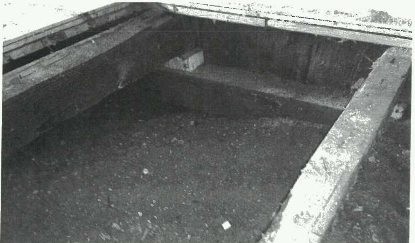
Figure 16. No solid blocking between floor joists
