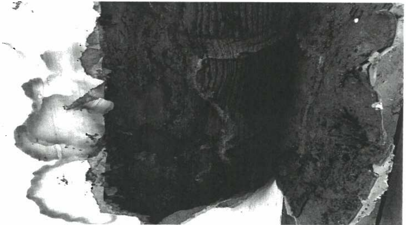
Figure 6. Heavy termite infestation and damage at partition boards.
