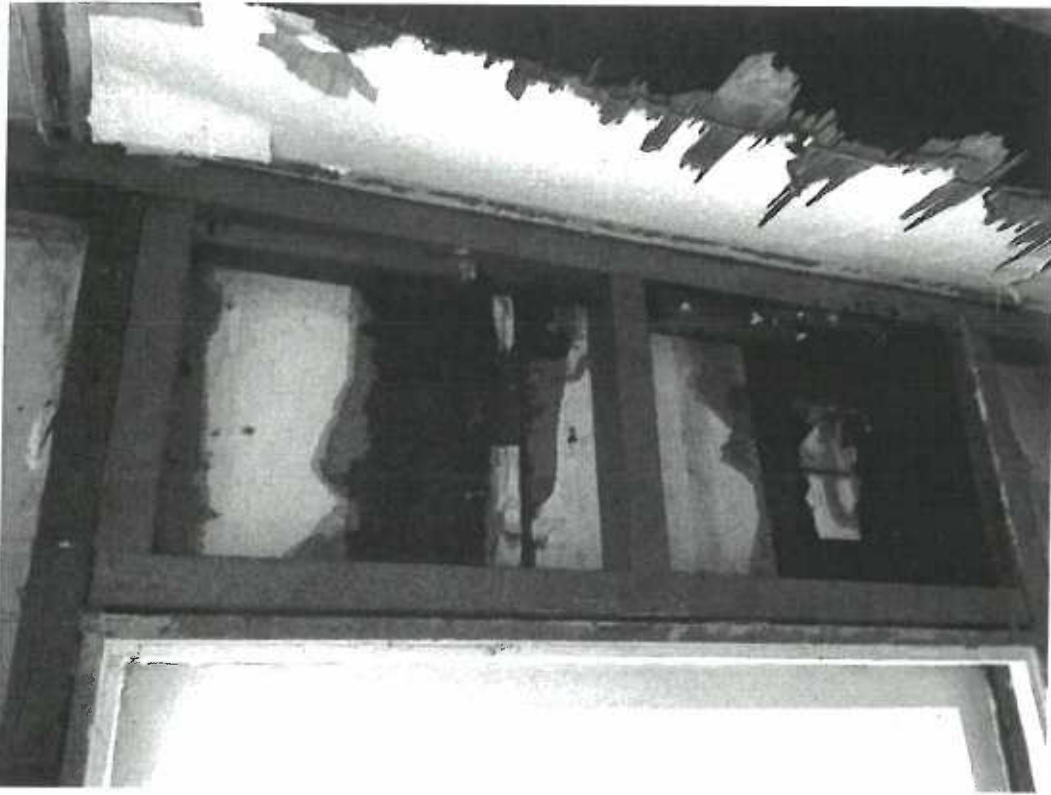
Figure 7. Place holder Sub-standard door and window framing
