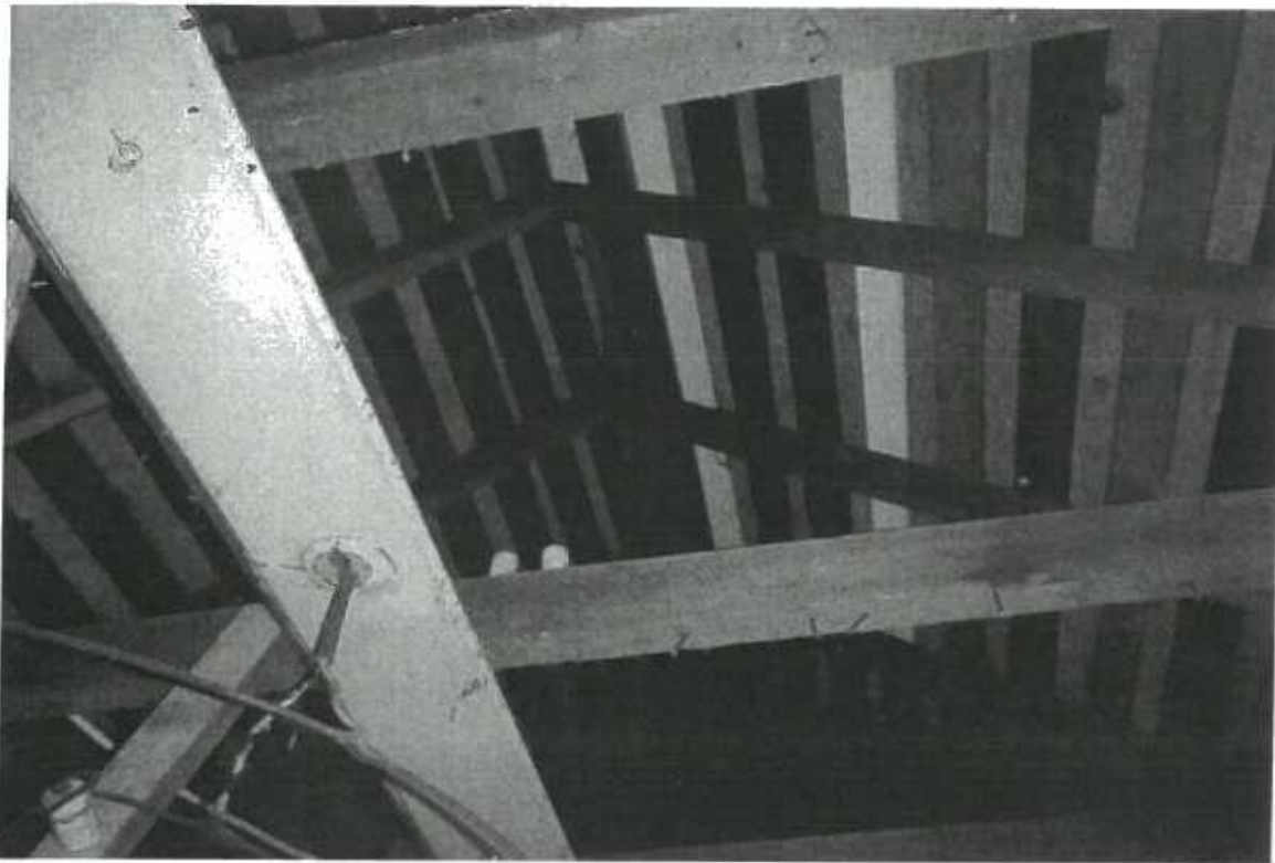
Figure 1. Roof framing, no ridge support, solid blocking
