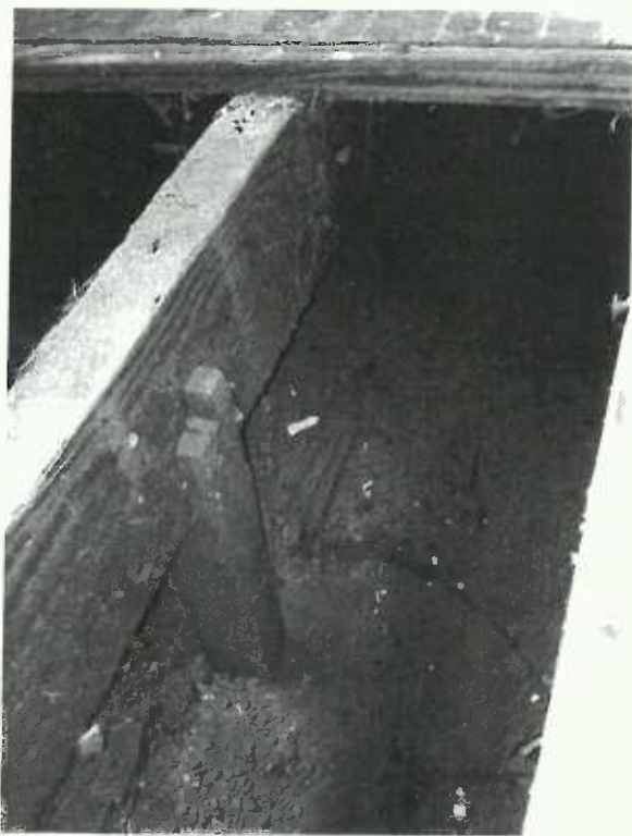
Figure 14. Posts bearing on soil alone
