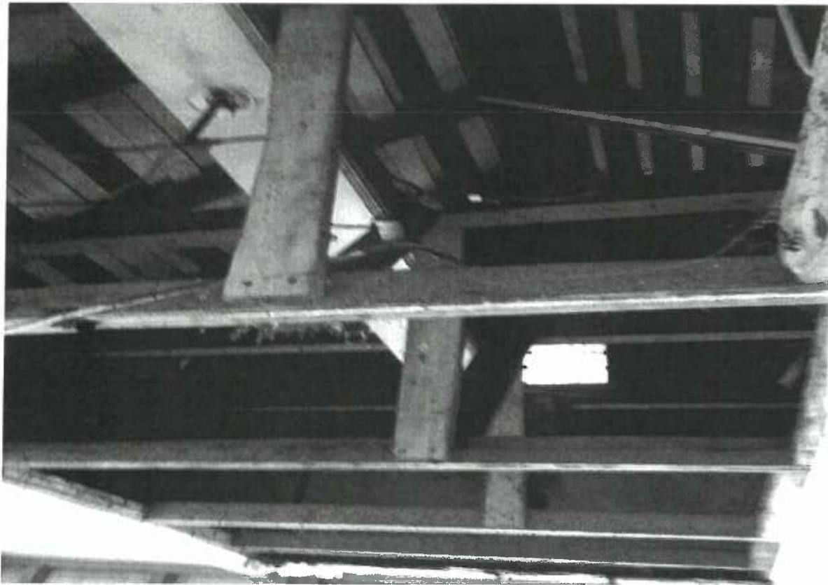
Figure 4. No wall framing at lines of bearing
