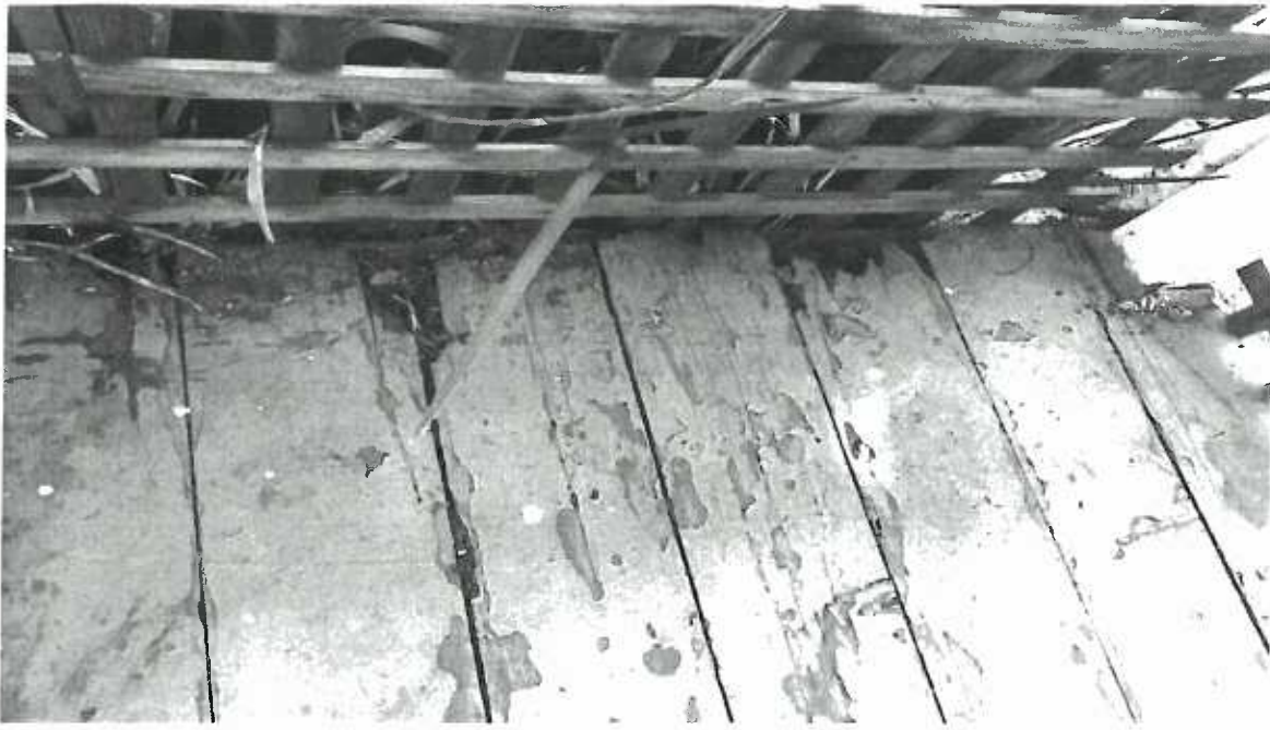
Figure 17. Porch deck shows heavy damage
