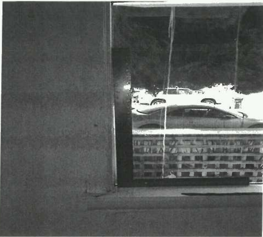
Figure 15. Front wall showing significant racking/shift towards SW corner
