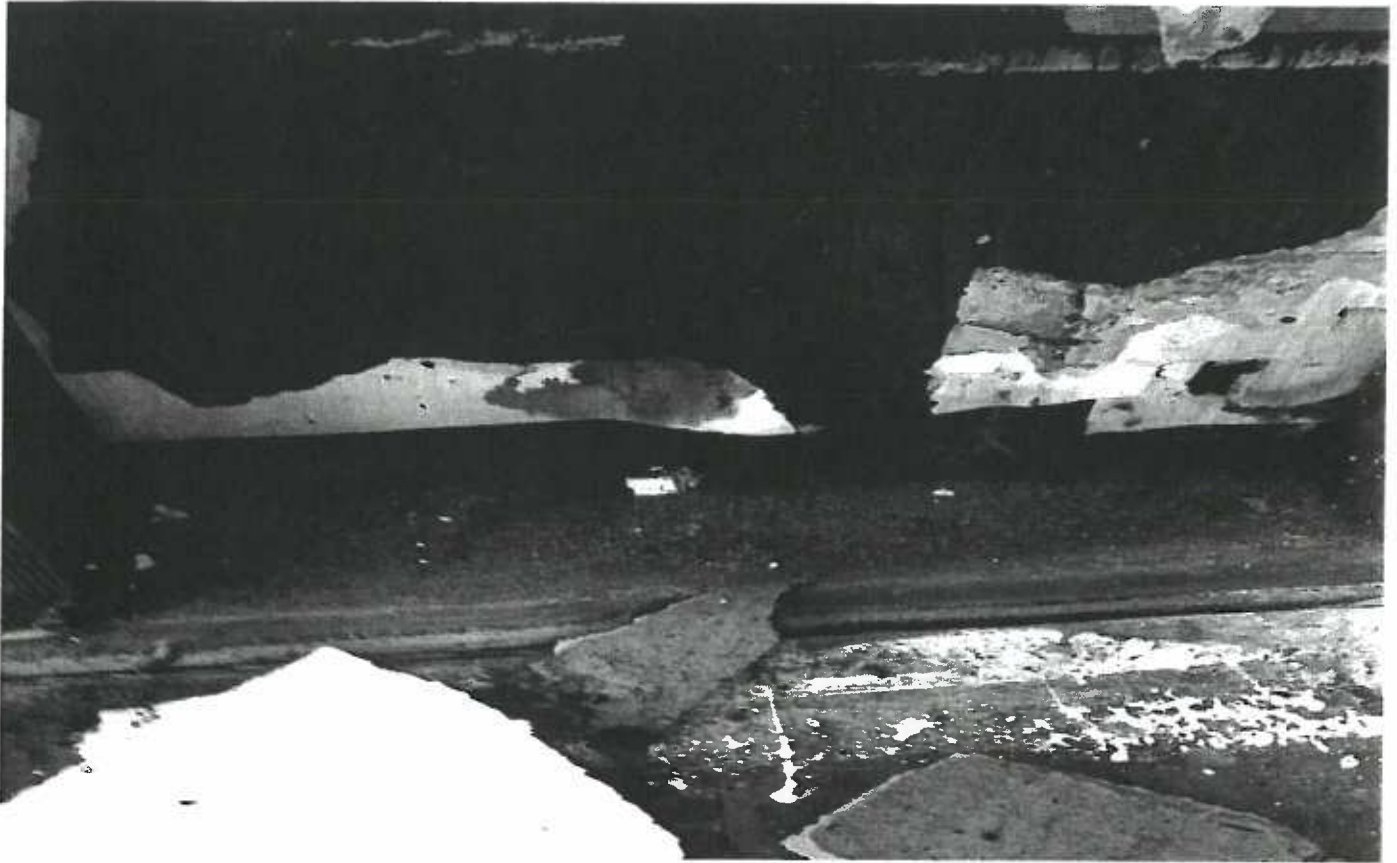
Figure 5. Heavy termite damage and infestation at partition boards
