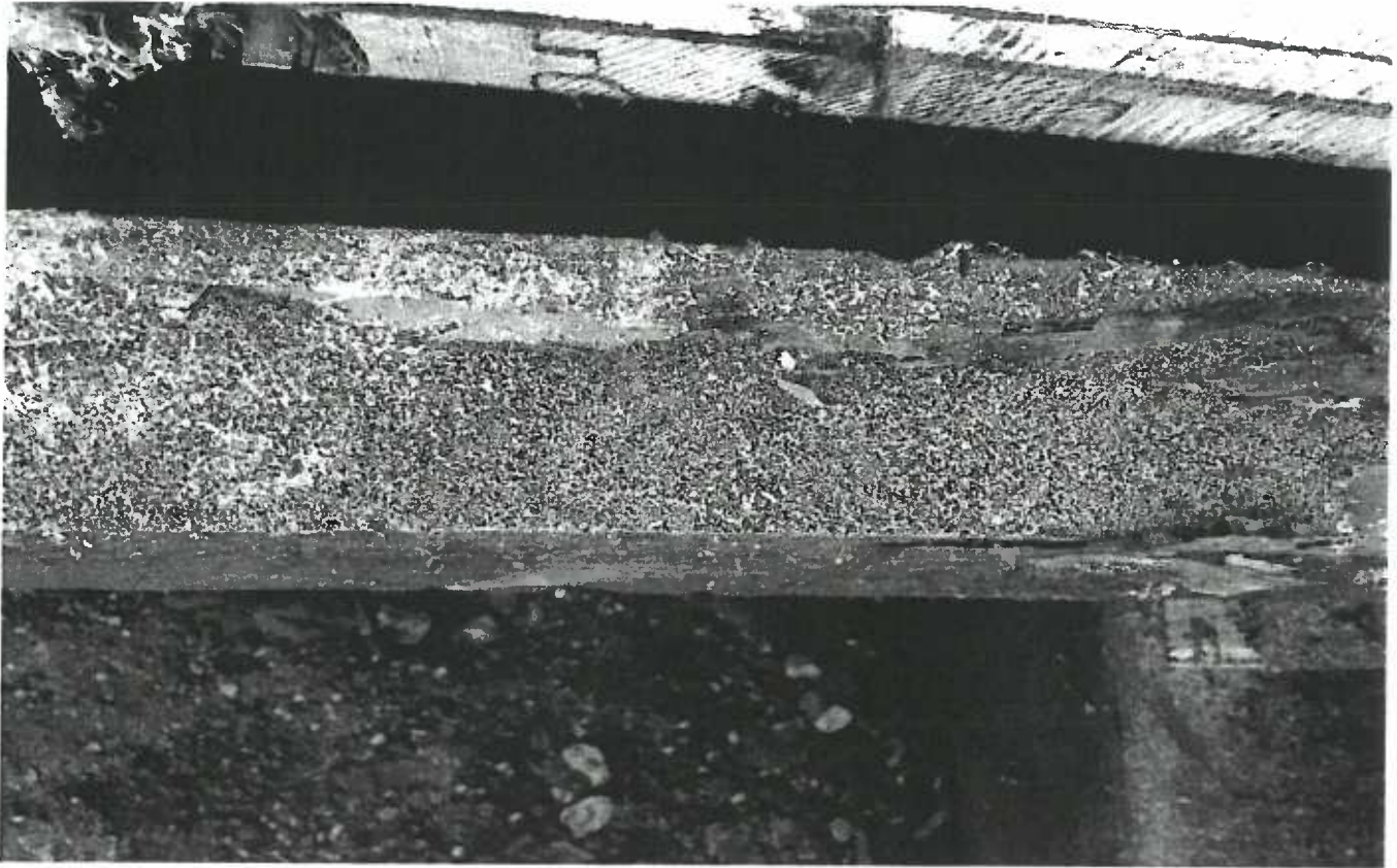
Figure 11. Heavy termite infestation and damage at floor joists
