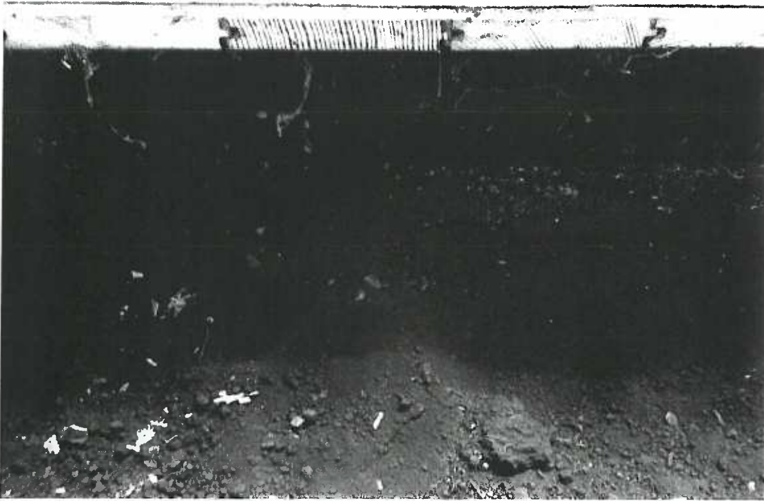
Figure 9. Mudsill completely embedded into soil
