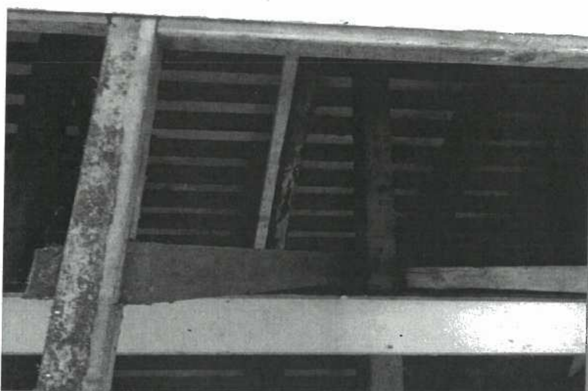
Figure 2. Heavy Termite infestation and damage at rafters
