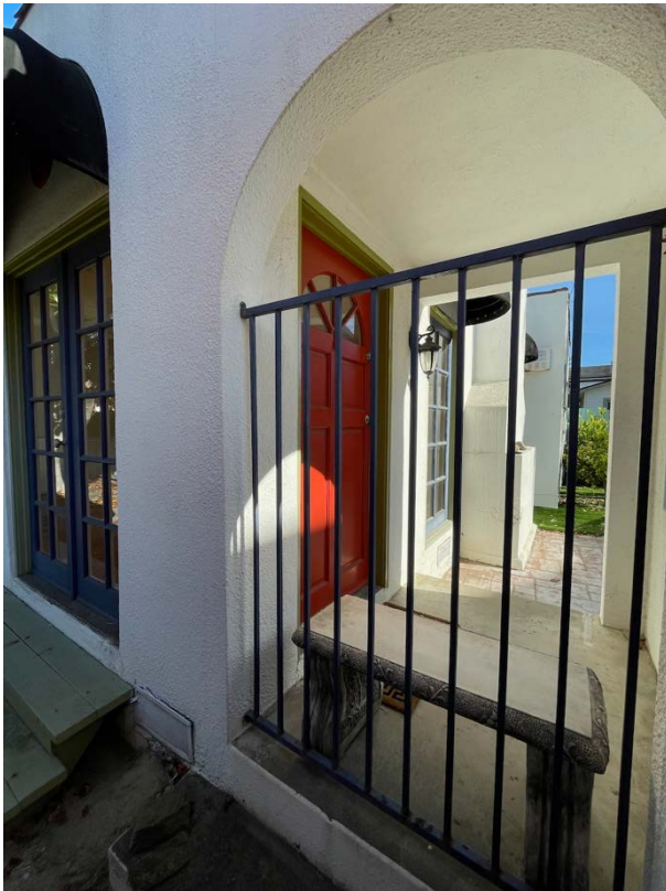
Figure 7. Front (northwest) elevation, concrete steps to porch blocked by metal railing; replacement front door. (Source: Site visit, December 5, 2023).
