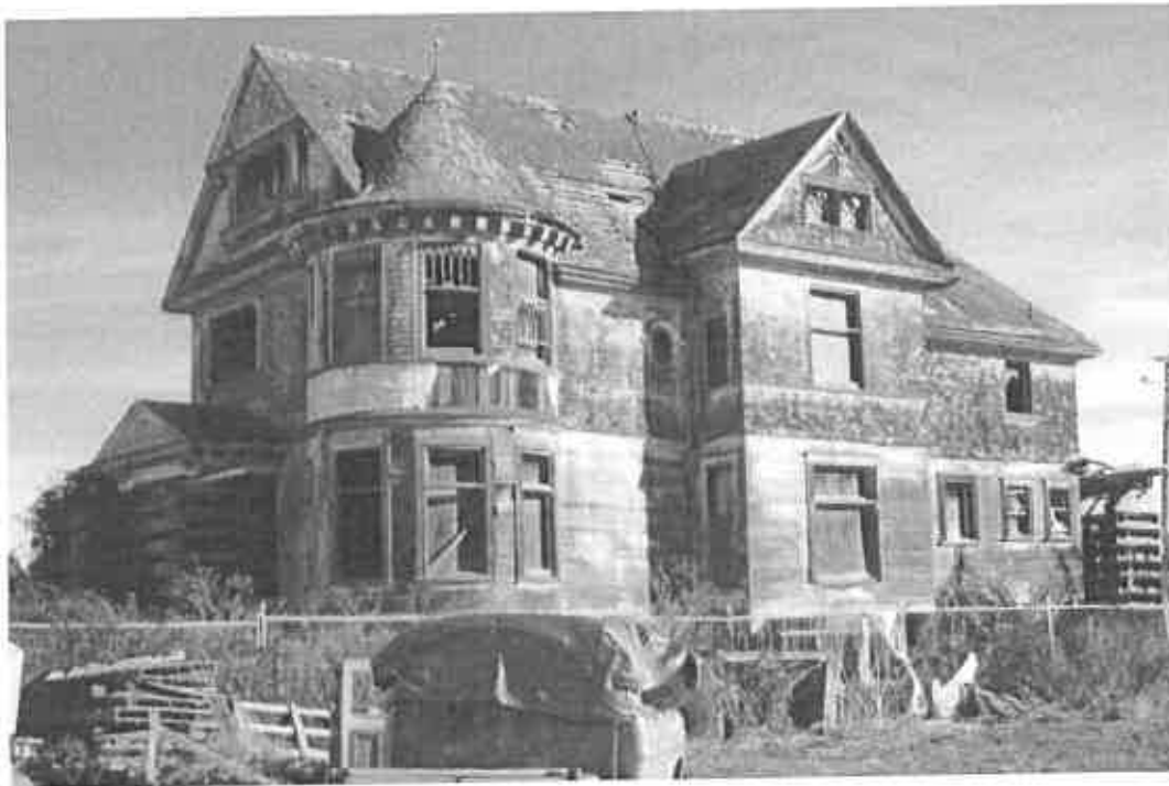
Photo #2. Looking SE at West side-elev., note deterioration of build. materials, & loss of decorative components. Kent Seavey, December 29, 2024.
