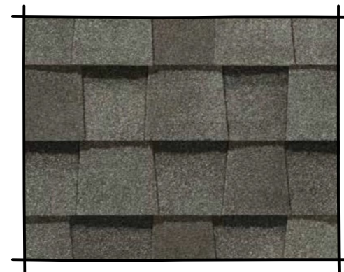
EXISTING COMPOSITION SHINGLE TILE ROOF
