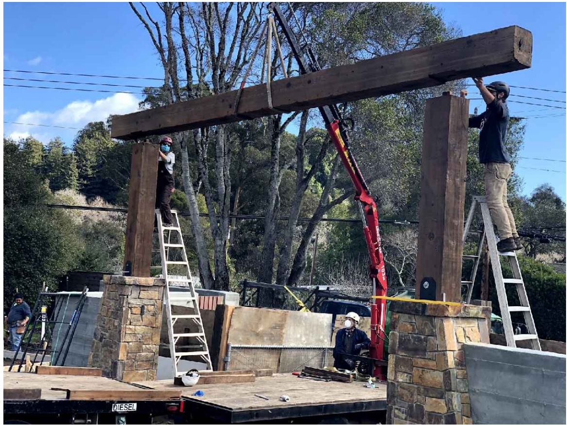
TIMBER FRAME LET-IN LAP JOINTS
