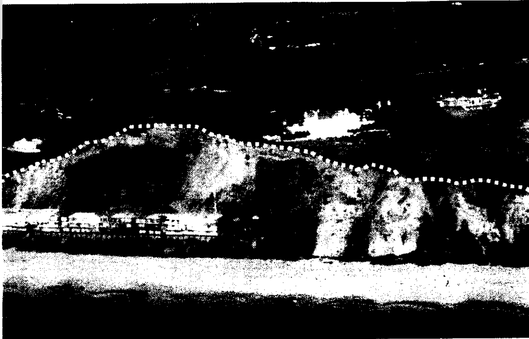
Figure 1. Bluff failure at Place de Mer, ~ 1000 feet upcoast from Sand Dollar Beach from the Loma Prieta earthquake. Yellow dotted line delineates top of slope failure. Red arrow points to a house that was demolished following the earthquake due to loss of support.
