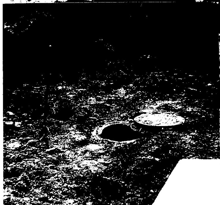
Grading To Find Manhole, Recomaction 1996 Sanitation Project Permit #96-0396
