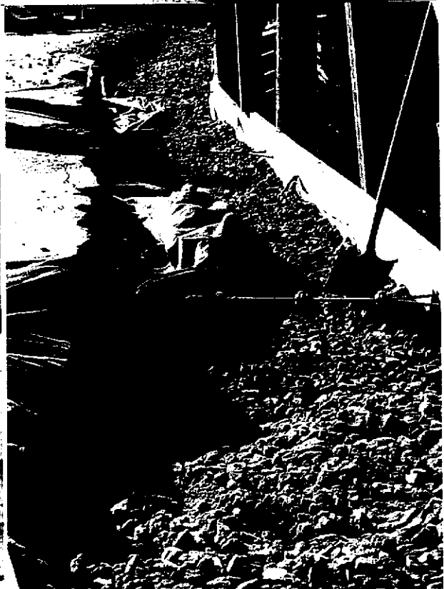
Concrete Grade Beam, Drain work, Drain Rock, Dead Men 1996 Sanitation Project Permit #96-0396
