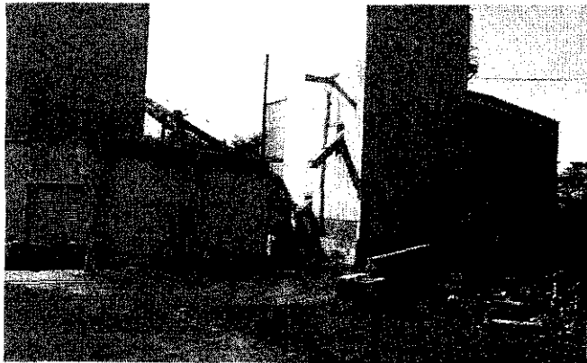
Existing northwest elevation of project area. Tall building at right center (with angled materials chute) is to be added to. One-story building at left center is to be demolished to accommodate footprint of proposed building addition.
