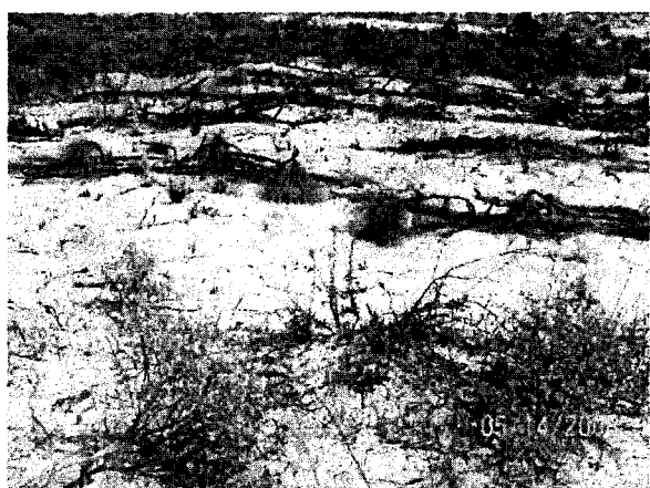
Figure 3: Example of dense planting with brush in upper zone of highwall. The limbs are well anchored to the slope. Middle and lower zones are in the background.
