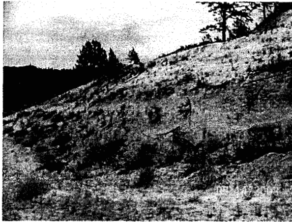
Figure 7: Area B dense planting with brush needs additional brush anchored to bare area of slope.
