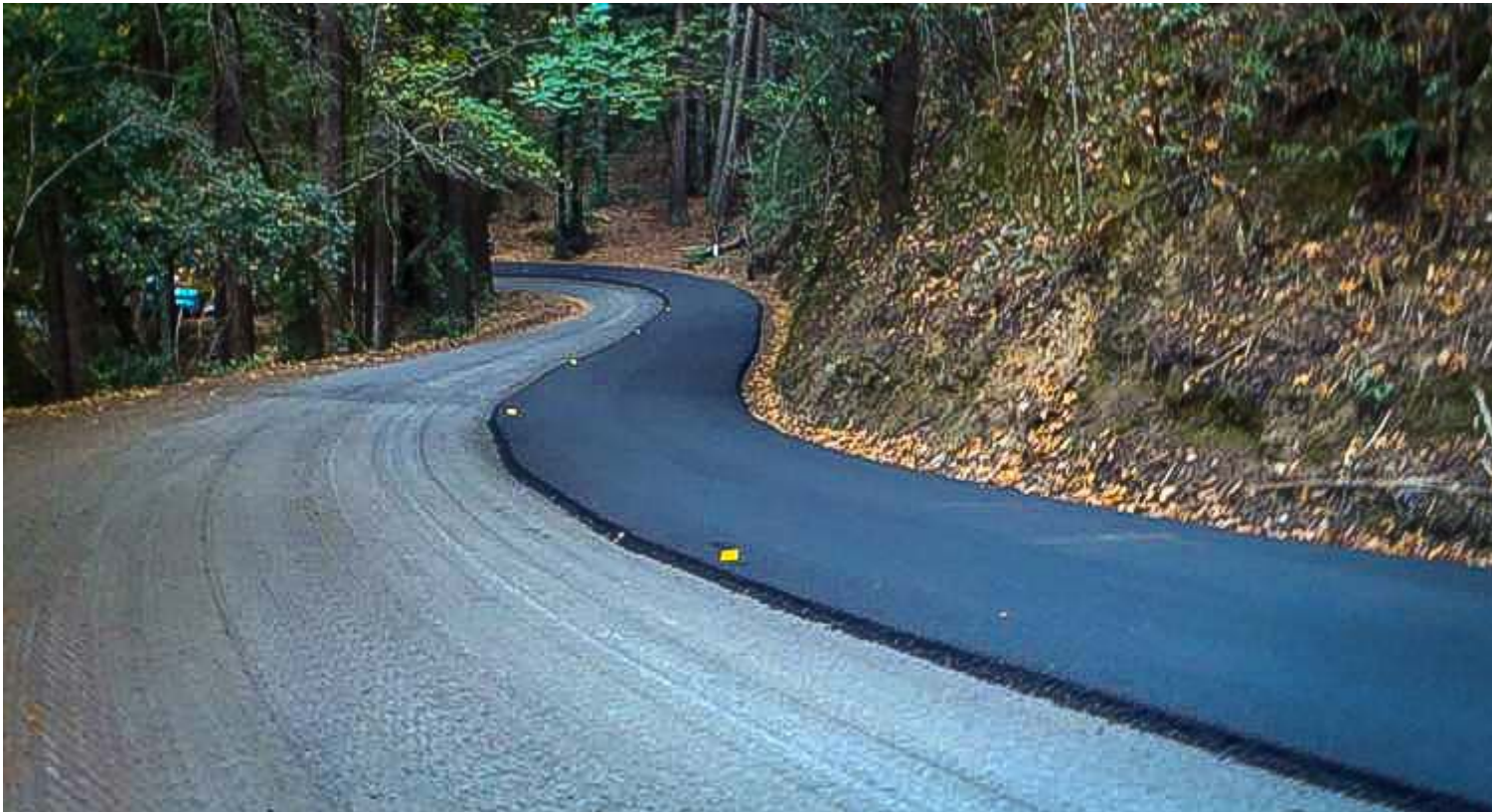
FELTON EMPIRE ROAD ASPHALT CONCRETE OVERLAY
