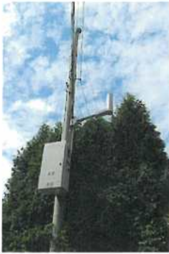
Microcell/Distributed Antenna System Node
