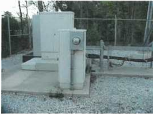
Cellular Base Station Ground Equipment
