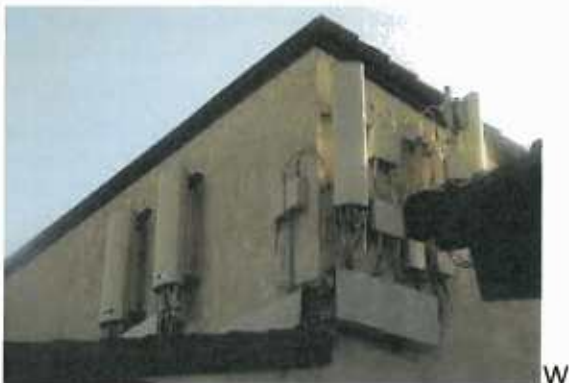
Wall Mounted Telecommunications Antenna System
