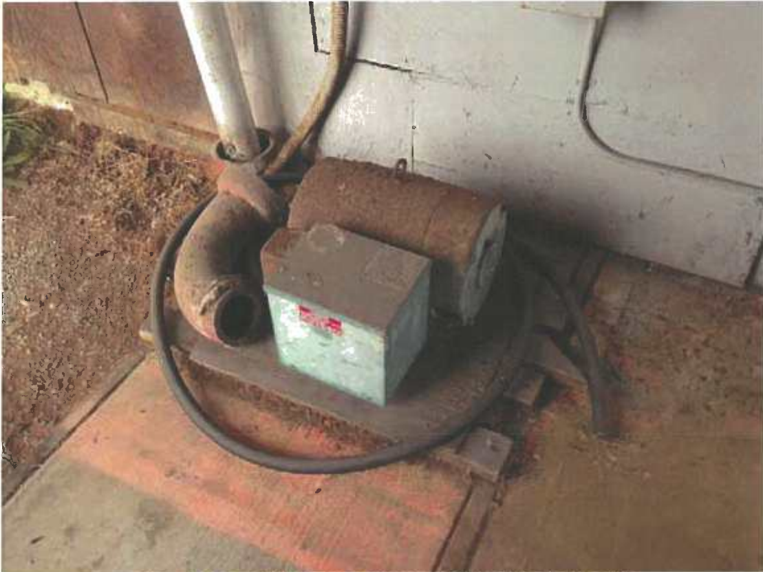
ROTARY PHASE GENERATOR ADJACENT TO WEST SIDE OF BUILDING
