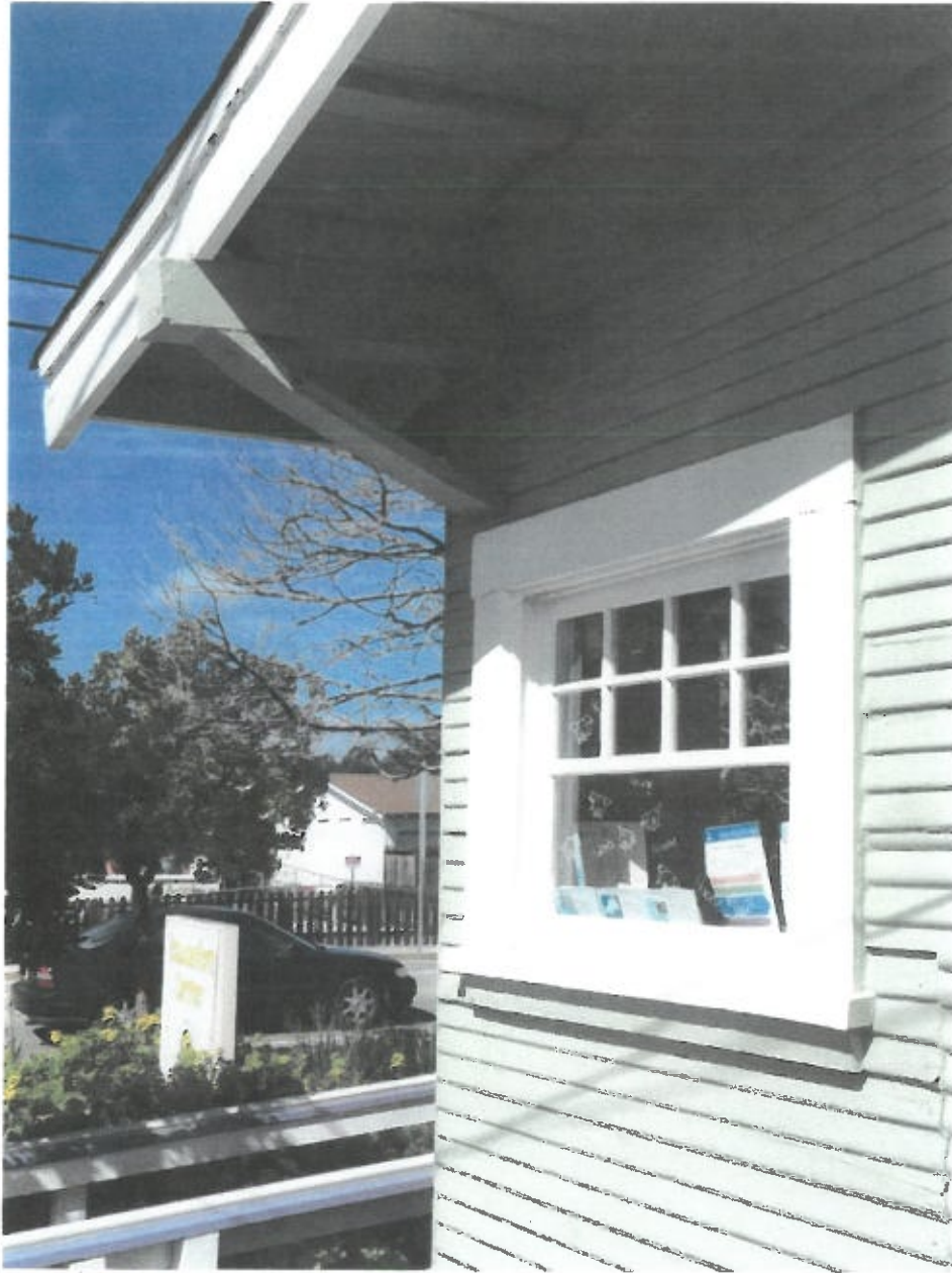
Outrigger bracket and window details at existing building. New work at training building will be similar.
