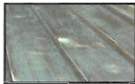
COPPER STANDING SEAM ROOF WITH PATINA
