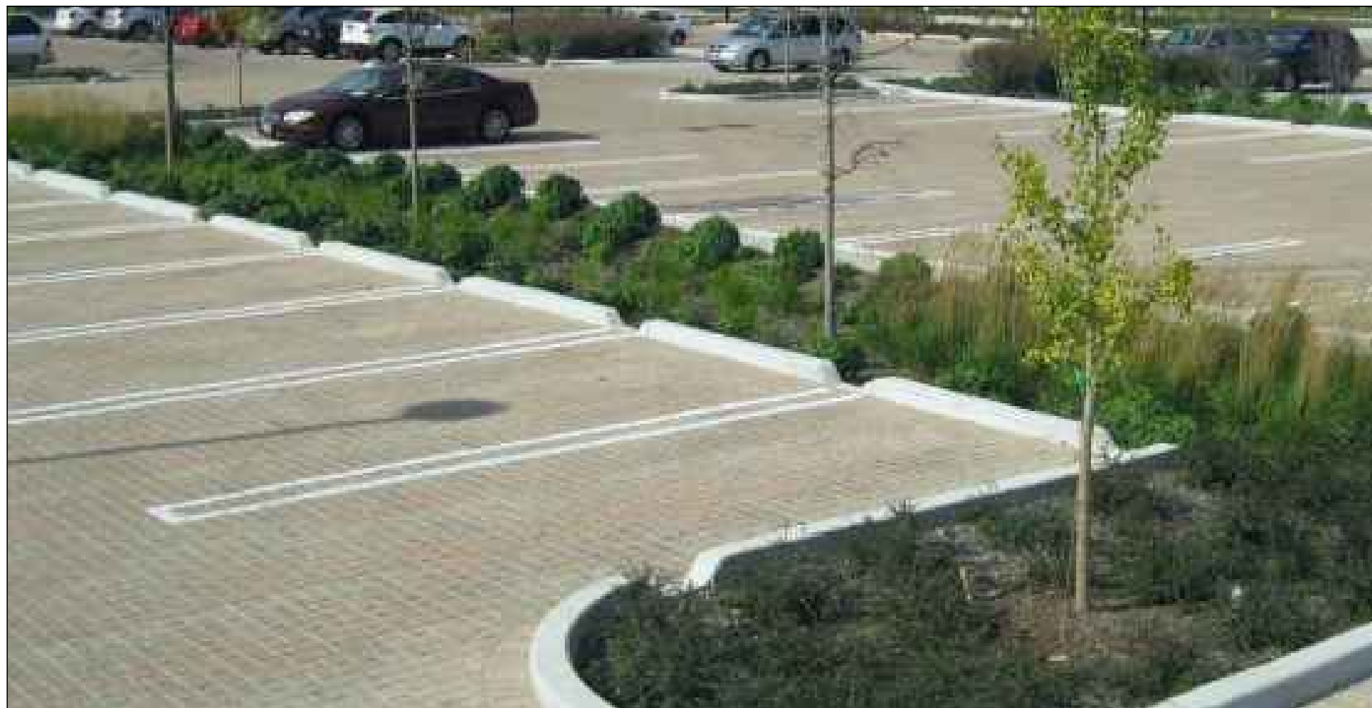
PARKING LOT WITH BIOSWALES TO TREAT ONSITE RUNOFF
