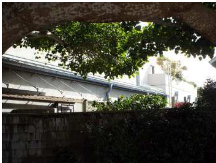
The second story setback is just above the rain gutter
