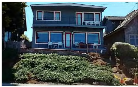
WEST ELEVATION - JULY 2023
