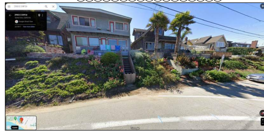
WEST ELEVATION - JULY 2023
