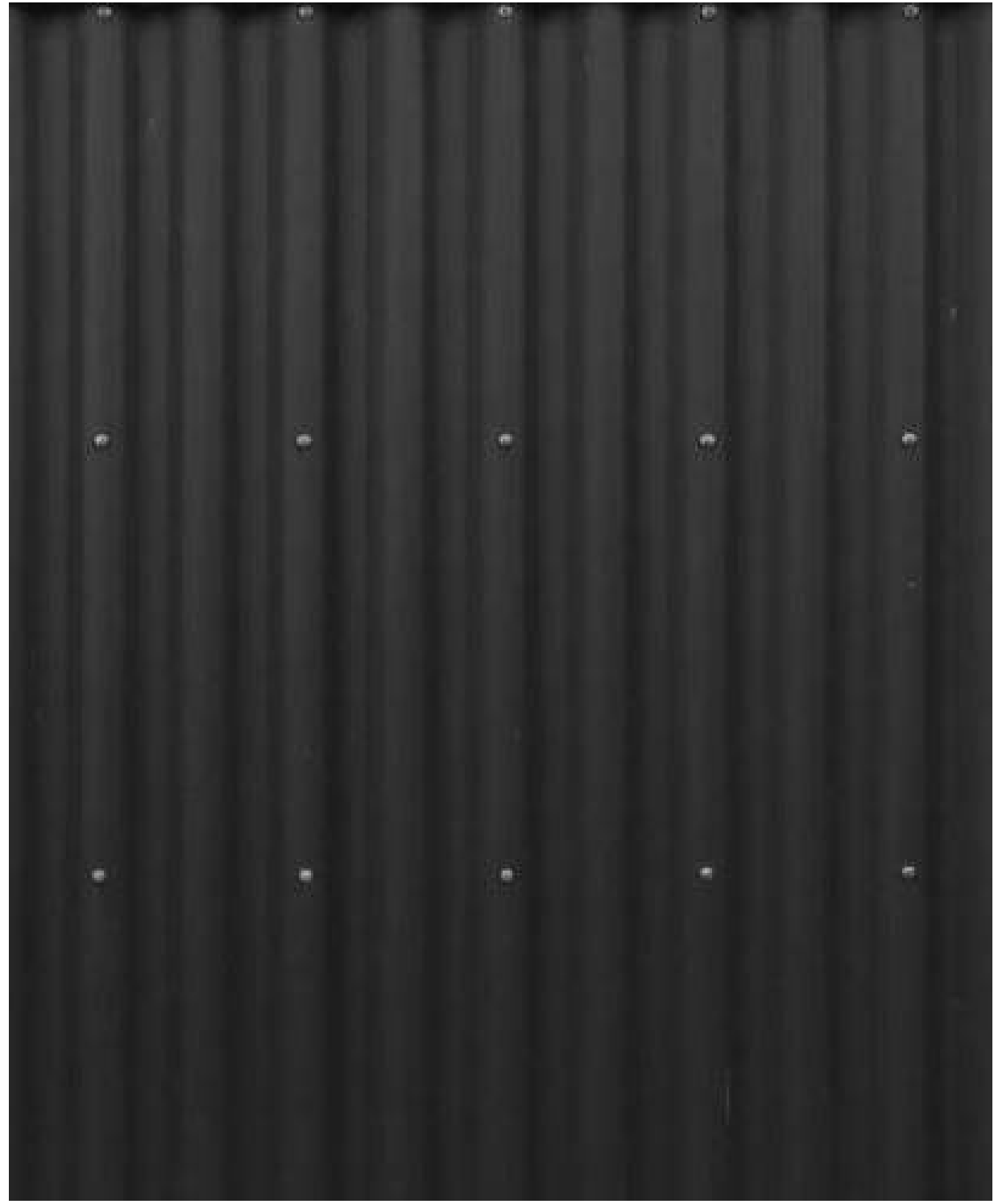
EXTERIOR PT'D DARK CORRUGATED METAL SIDING & ROOFING
