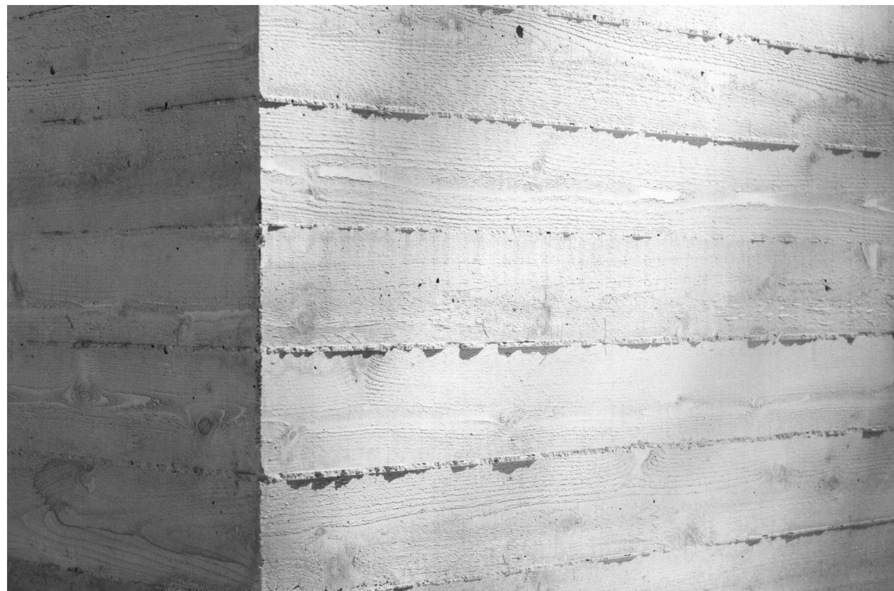
BOARD FORM CONCRETE SITE WALLS & EXPOSED FOUNDATIONS
