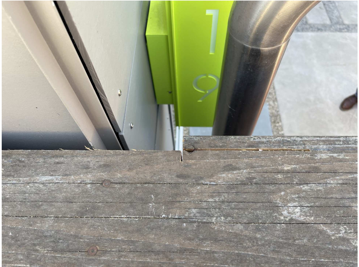
Showing how the Cap of my Fence was cut into so that Structure could eliminate even 1 inch of Setback to Zero Inches
