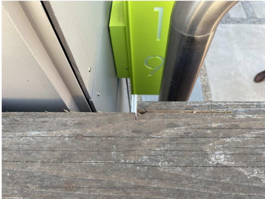
Exhibit C. The cap of the shared fence, notched to accommodate the wall of the structure.
