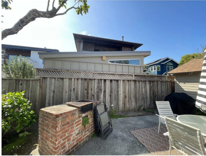
Exhibit A. View from the rear yard of 145 18th Avenue. The structure stands above the shared fence, with a window above the fence line looking into the yard. The shade it casts is visible across the yard.
