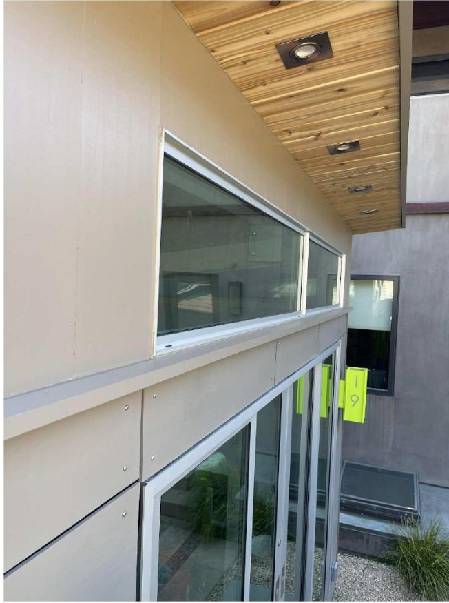
Exhibit F. Windows and sliding glass doors in the wall facing the residence, and the glazing at grade on the residence visible at right — the light well discussed in Section VIII.
