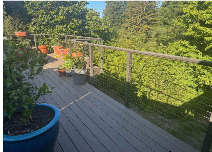
① VIEW TOWARD PROPERTY LINE
