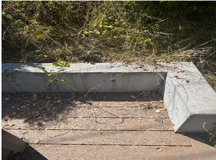
③ VIEW OF RETAINING WALL
