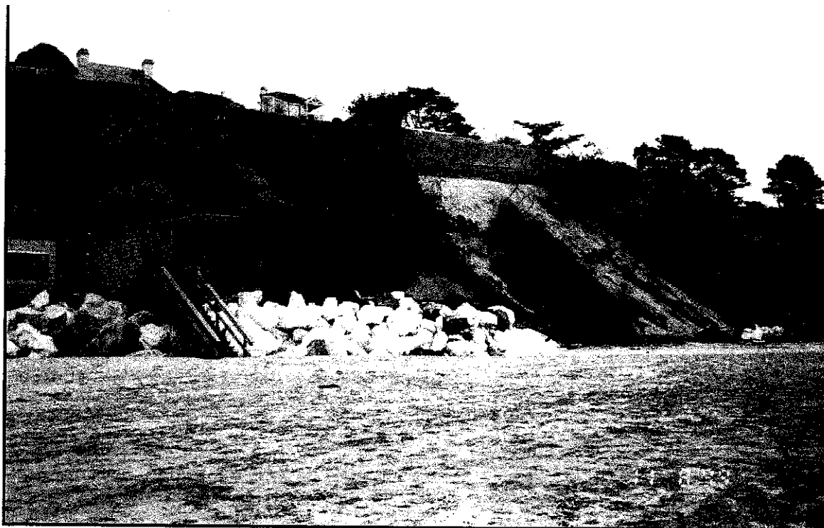
Photograph of the bluff approximately 1,500 feet north of the Curtis property. This photograph was taken immediately following completion (1999) of a reinforced shotcrete wall along the upper 20 feet of the bluff. The shotcrete has been stained to mimic the natural color of the earth materials in this area. Notice the soldier beam and lagging retaining wall to the north of the shotcrete face. View to northeast.
