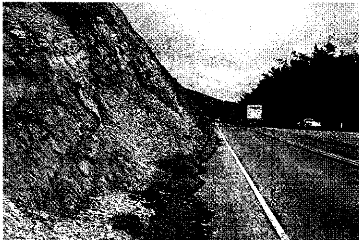
This view shows the existing inadequate rock catchment area, shoulder area, and bicycle lane now present at the toe of the rock slope which is to be cut back
