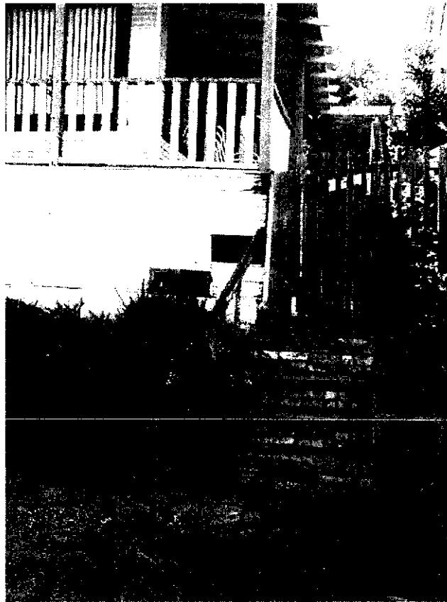
Figure 3. View of existing entry steps and dry rot at porch
