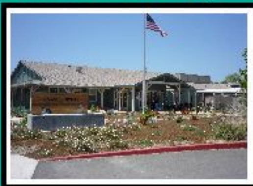
Animal Services Facility
