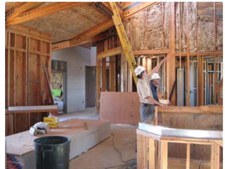
Interior of the Live Oak Resource Center during construction
